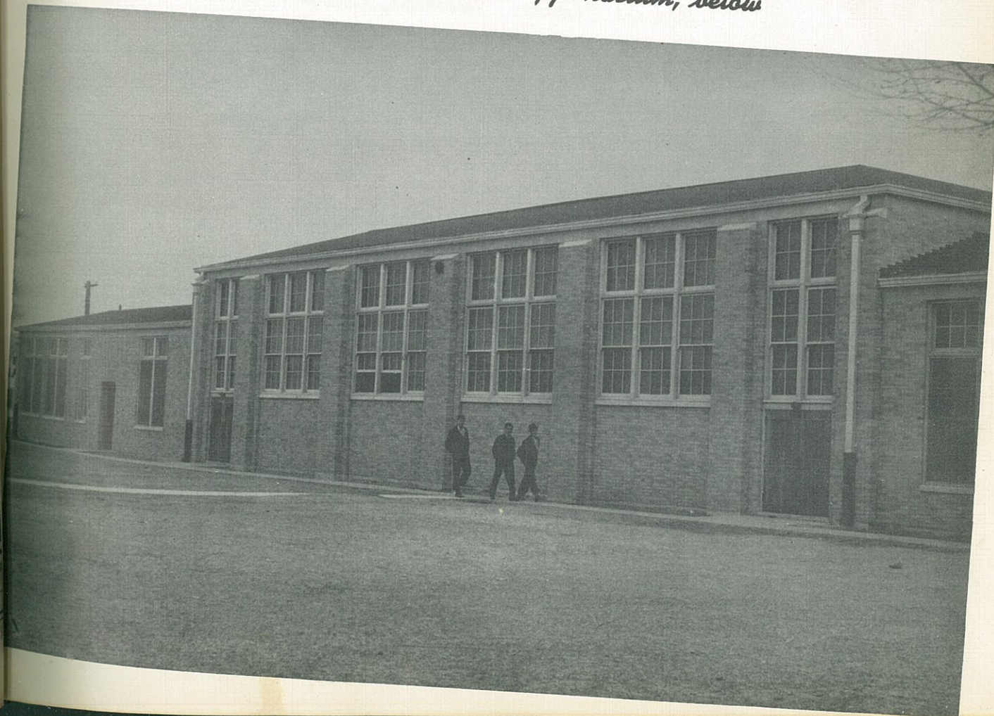
Field House, above; Gymnasium, below
